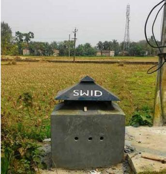
FIGURE 4.1: A) WATER LEVEL RECORDERS INSTALLED IN MULTIPLE AQUIFERS (LEFT); B) THE SECURED STRUCTURE FOR TELEMETRY DESIGNED BY THE STATE WATER INVESTIGATION DIRECTORATE, GOVERNMENT OF WEST BENGAL (RIGHT)
