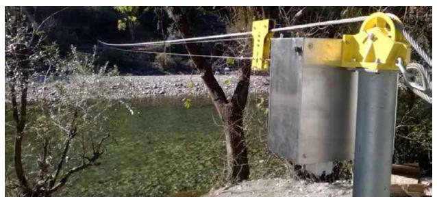
FIGURE 3.23 (A): AN AUTOMATIC CABLEWAY INSTALLED ON BEAS RIVER IN HIMACHAL PRADESH
