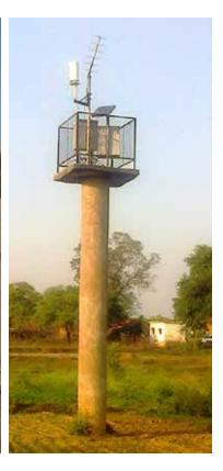
FIGURE 3.16: EXAMPLES OF GAUGE HUTS FOR WATER-LEVEL MONITORING SITES: A) A MASONRY HUT ON A RIVER BANK IN MAHARASHTRA; B) A STEEL ENCLOSURE ON A BRIDGE, GUJARAT; C) A PILLAR ERECTED FOR PROTECTION OF EQUIPMENT BY CWC IN ODISHA
